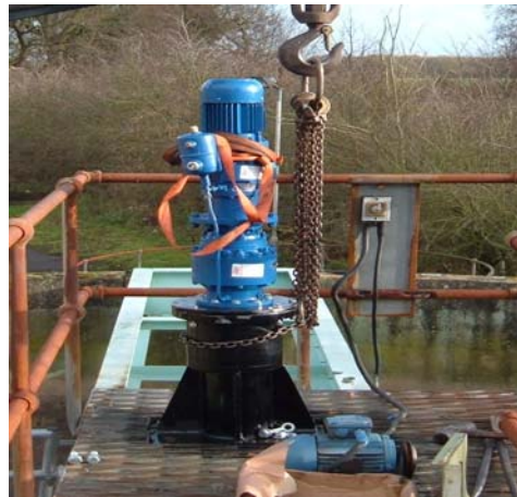
Brevini gearbox mounted onto bell housing
